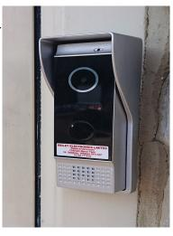
The camera can be fitted viewing straight ahead or at an angle on an angled plate to allow better visibility, the system has a 2 way speech channel so you may communicate with the visitor with ease.
